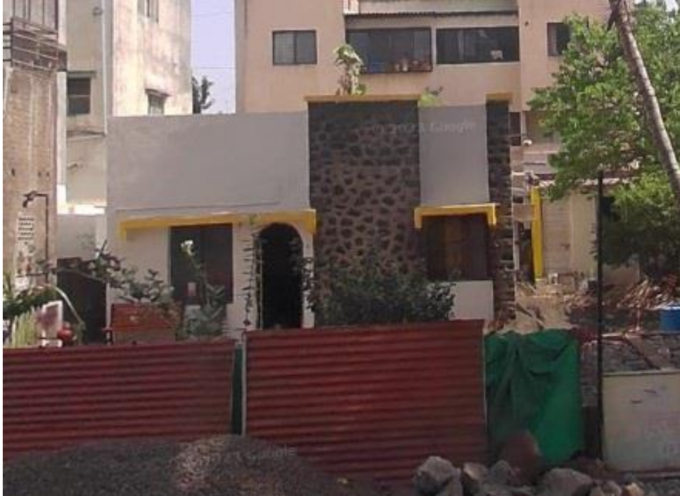
OFFICE BUILDING UNDER CONSTRUCTION (NORTH ELEVATION)
