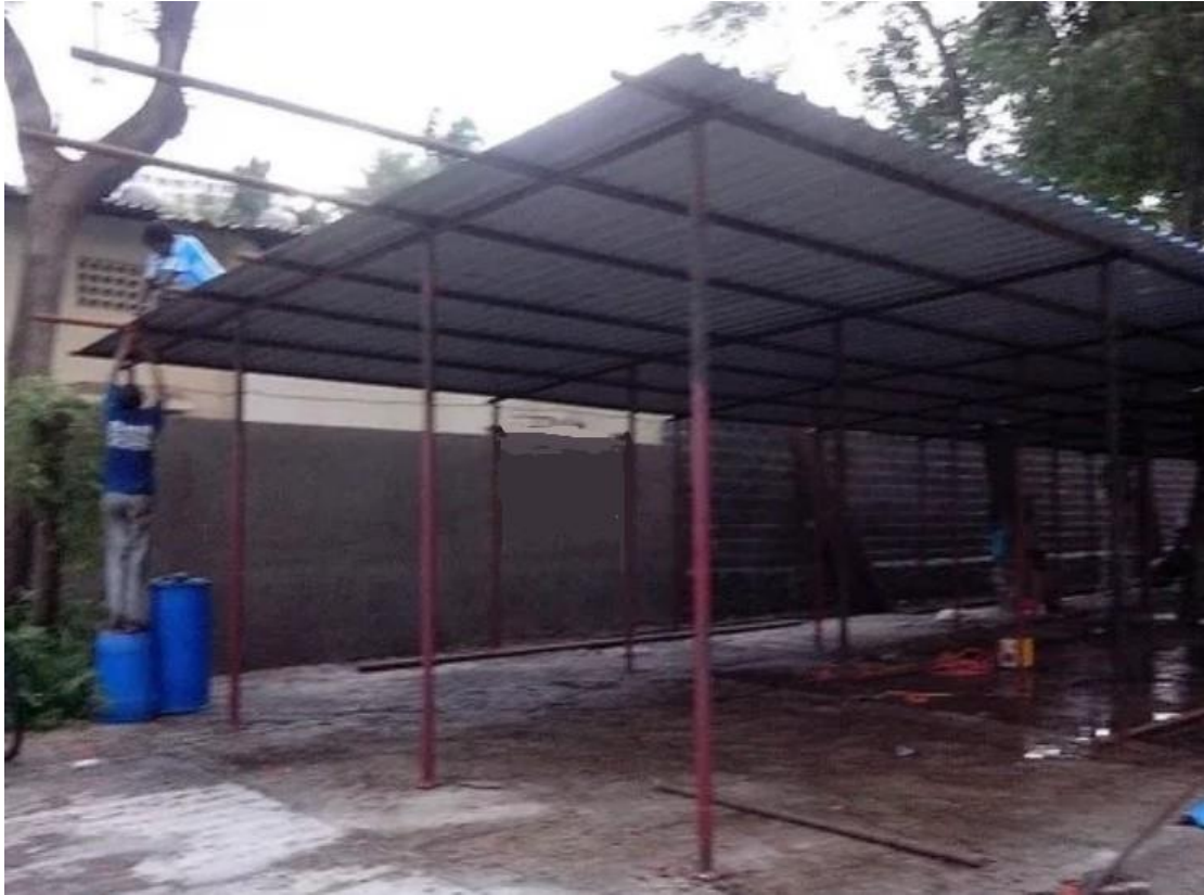
PARKING SHED UNDER CONSTRUCTION
