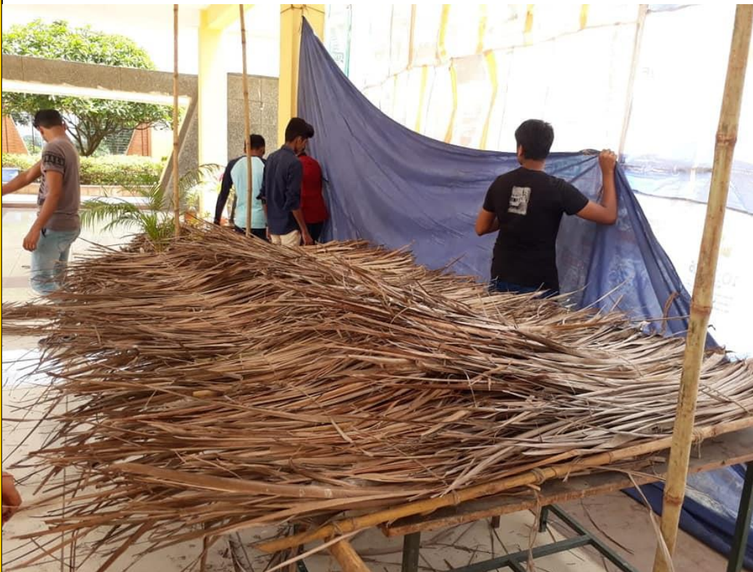
Thatched is used as a roofing material
