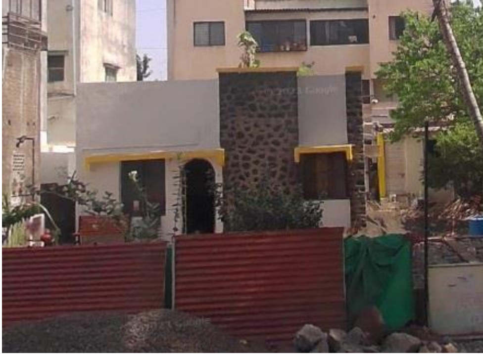
OFFICE BUILDING UNDER CONSTRUCTION (NORTH ELEVATION)
