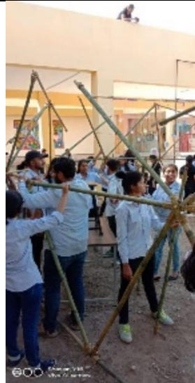
Students working on geodesic dome Joinery
