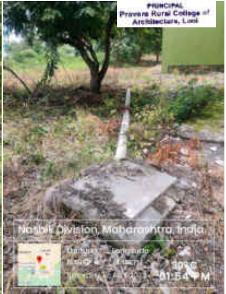
Liquid waste from toilets is channeled through pipes into soak pits
