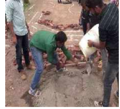
Students preparing mortar to construct masonry wall at the garden site
