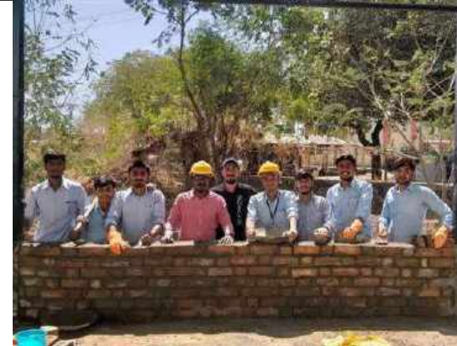
Brick masonry wall in double Flemish bond prepared by students at construction courtyard
