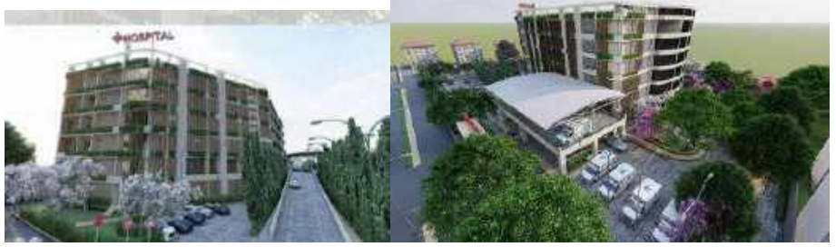
Final Views of Hospital Project
