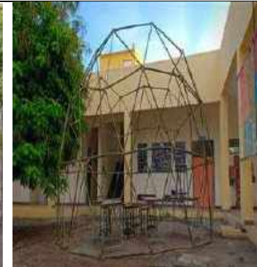
Geodesic Dome of 9M Diameter prepared by college students
