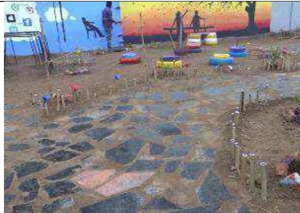
Pathways prepped from the recycled material (Waste tiles)
