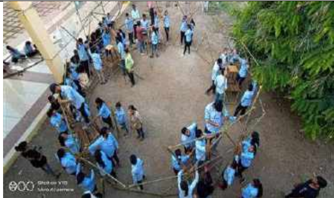
Students working on Bamboo Geodesic Dome of 9M Diameter
