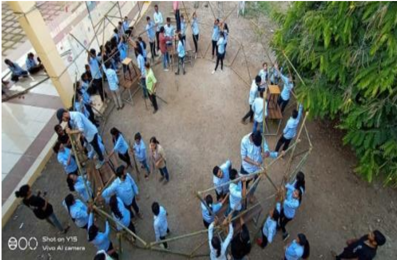
1.students working on geodesic dome
