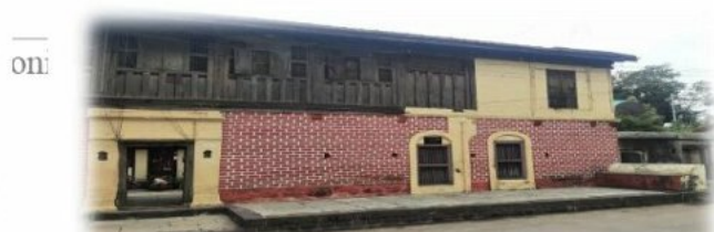
Fig 7: front view of front facade and side view of front facade
