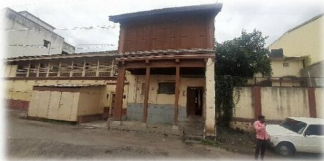
Fig 11: view of front façade
