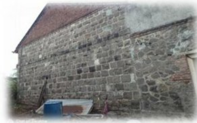
Fig 12: view of wall
