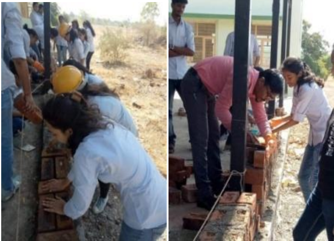
Faculty guide students about the actual execution of brick bonds construction.
