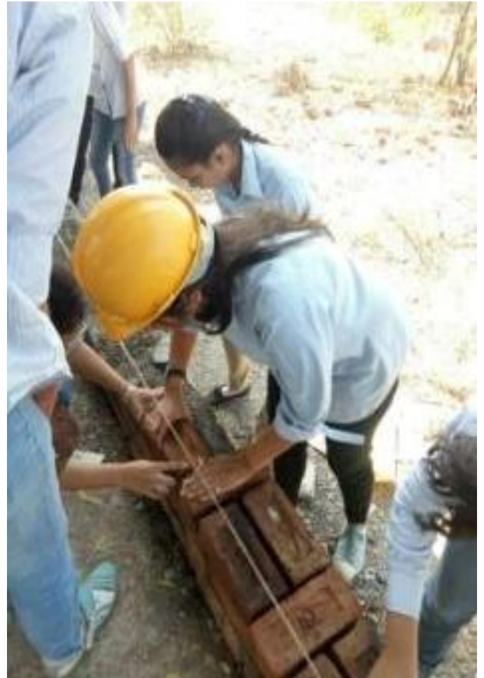
Students working on brick bond construction.
