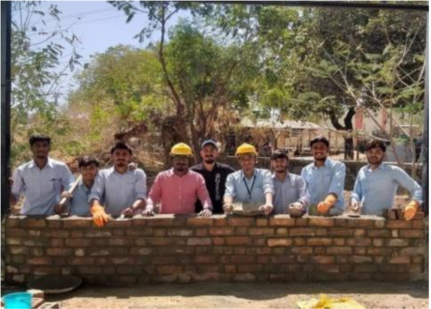
Under the guidance of faculty student completed the brick bond construction.
