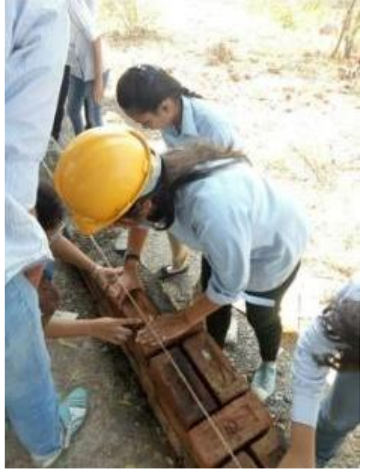
Students working on brick bond construction.
