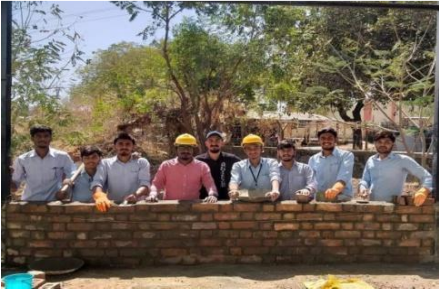
Under the guidance of faculty student completed the brick bond construction.
