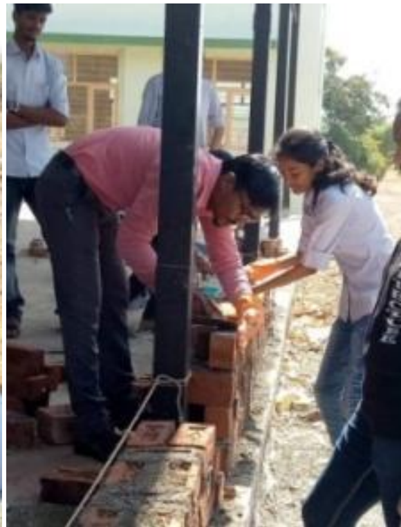
Faculty guide students about the actual execution of brick bonds construction.
