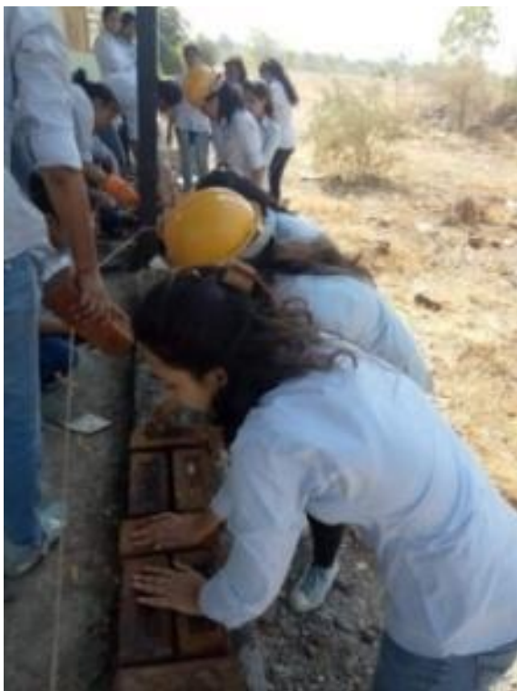
Faculty guide students about the actual execution of brick bonds construction.
