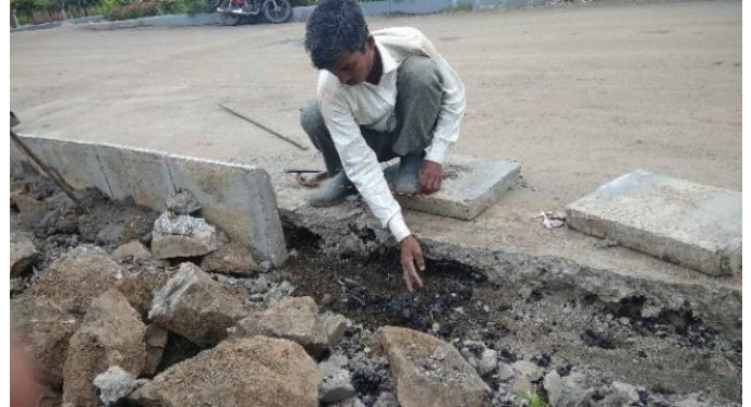
4 Ongoing Curb fixing as a edge to road on site
