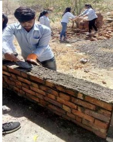
Students placing mortar for the next course of the brick wall in Double Flemish Bond
