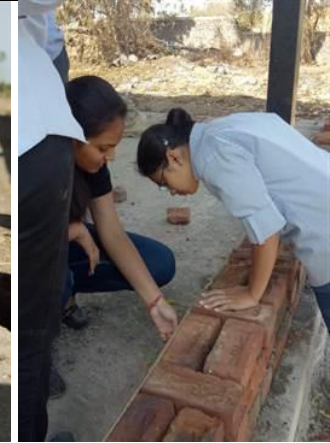
Students preparing mortar mixture and checking alignment of bricks to construct masonry brick wall
