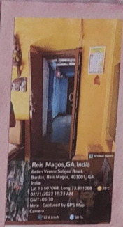
DOOR DETAIL OF WADA
