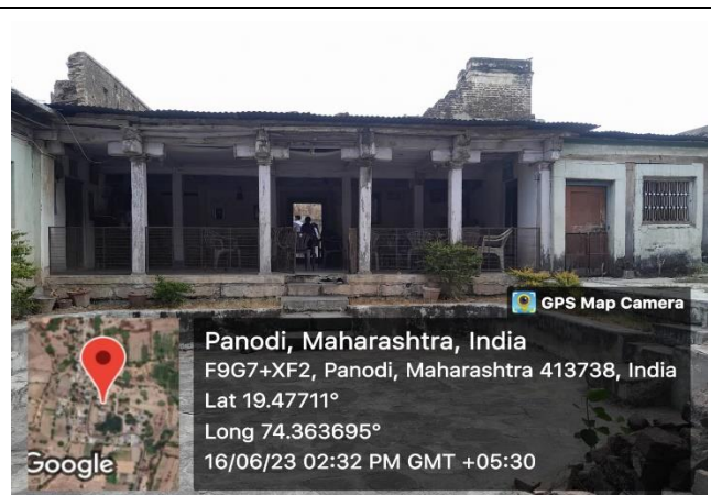
4.. Intact portion of wada
