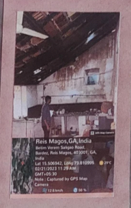
KITCHEN AREA OF WADA
