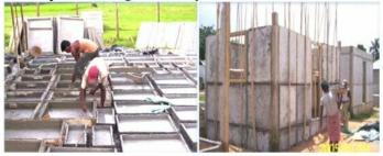
Figure 9: Ferro Cement Panels
