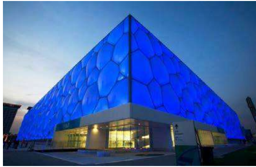
Figure 1. ETFE in facade of Beijing National Aquatics Center, Beijing, China
