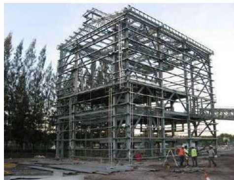
Figure 6:1: Steel structure installation
