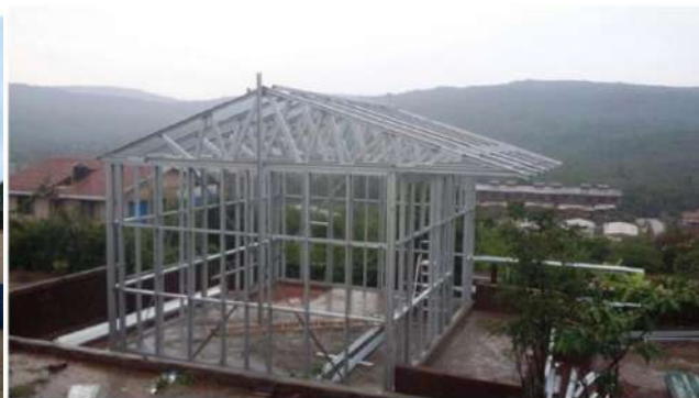
Figure 6:7 : Light gauge steel frame
