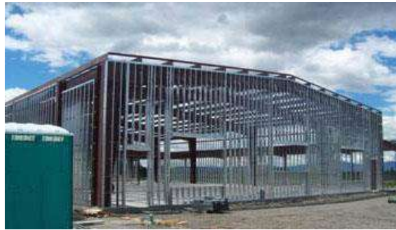
Figure 6:2 : Example of structural design for LGSF Construction
